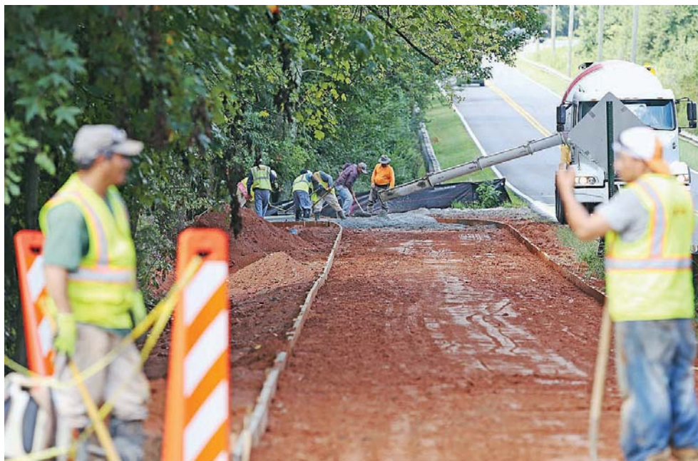
Pouring concrete near Kingsbridge Road.
